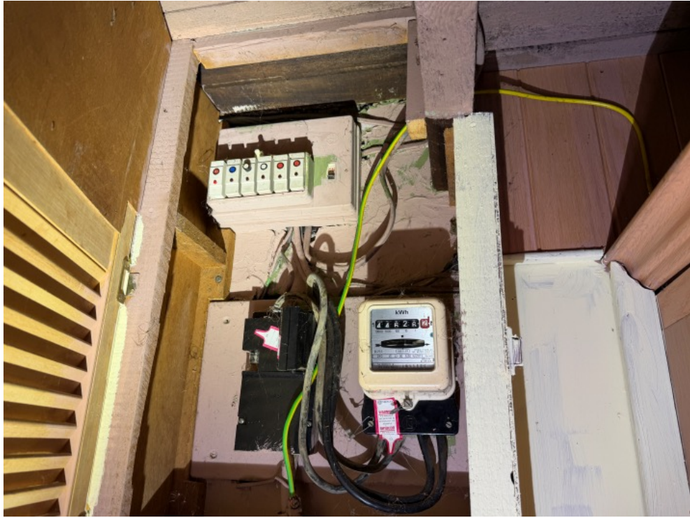
Electric meter and consumer unit
