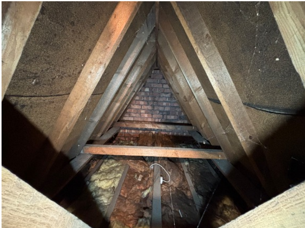
General view of roof structure
