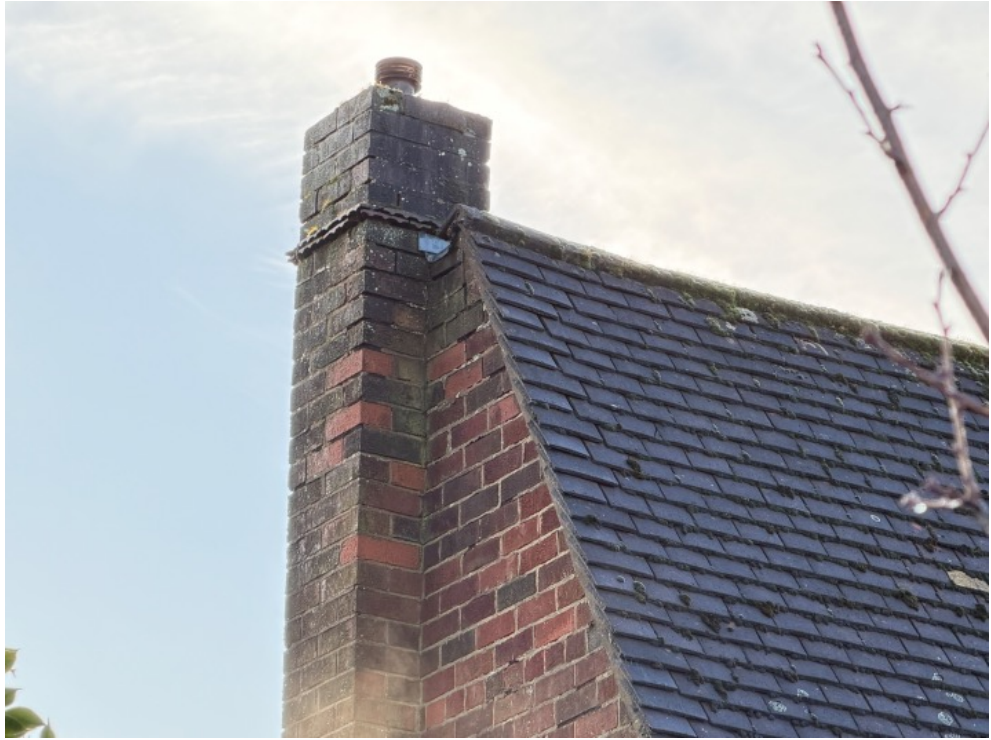
View of left side chimney
