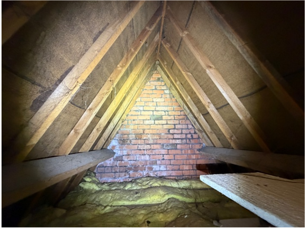
General view of roof structure
