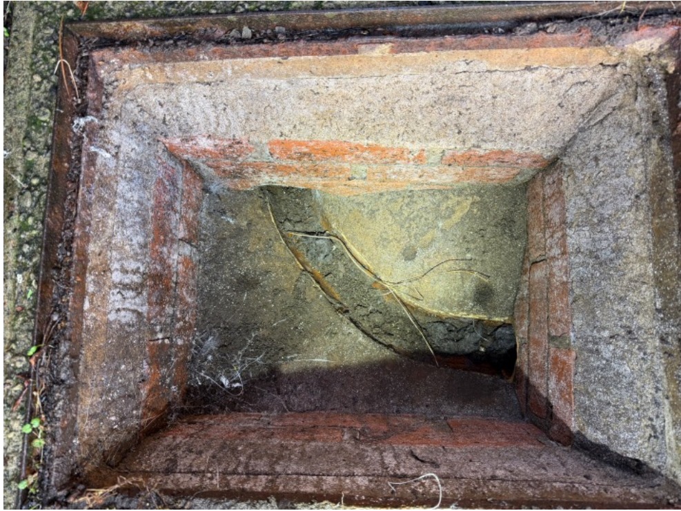
View down drain chamber
