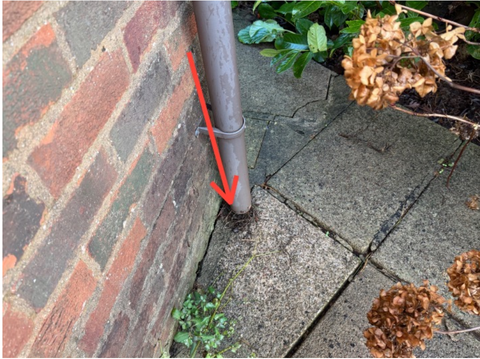
Rainwater downpipe to ground
