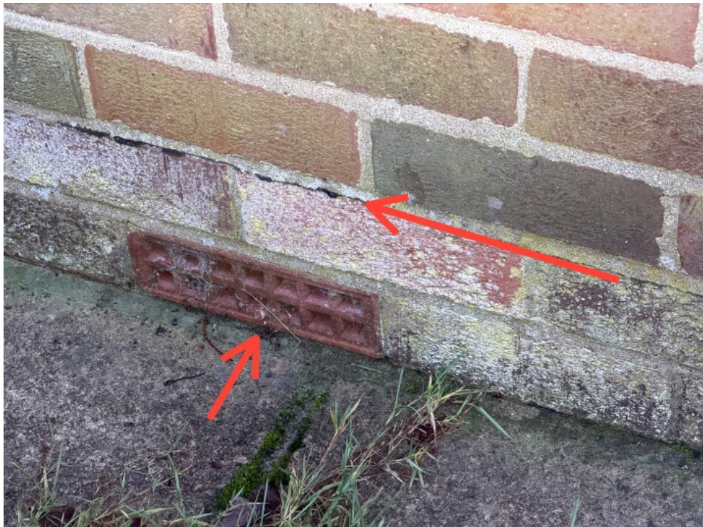
Subfloor ventilation points and dpc line - air brick in close proximity to ground level
